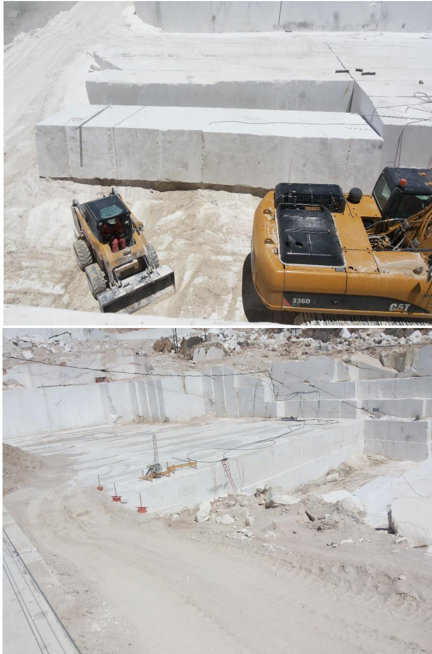
Figure 6: Marble Block removal
