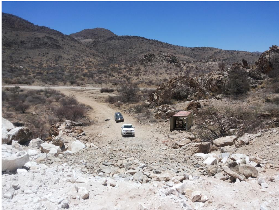
Figure 5: Typical new access road to an outcrop
