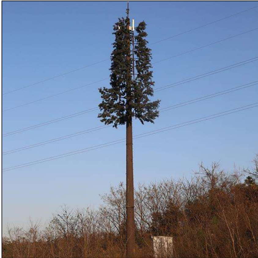
Figure 2: Example of a camouflaged tree telecommunication tower
