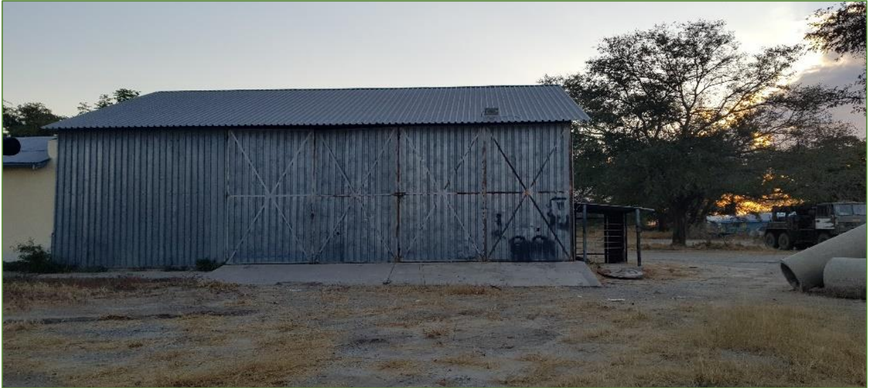
Figure 8: Existing RCC Workshop on site
