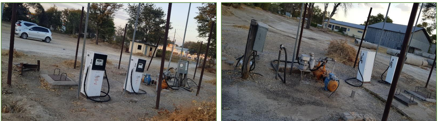
Figure 7: Existing RCC Underground Tanks on site
