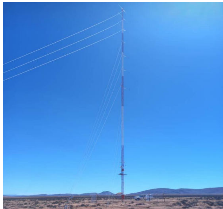
Fig 1: Show Rosh Pinah Wind Mast as installed on-site during quarterly maintenance.
