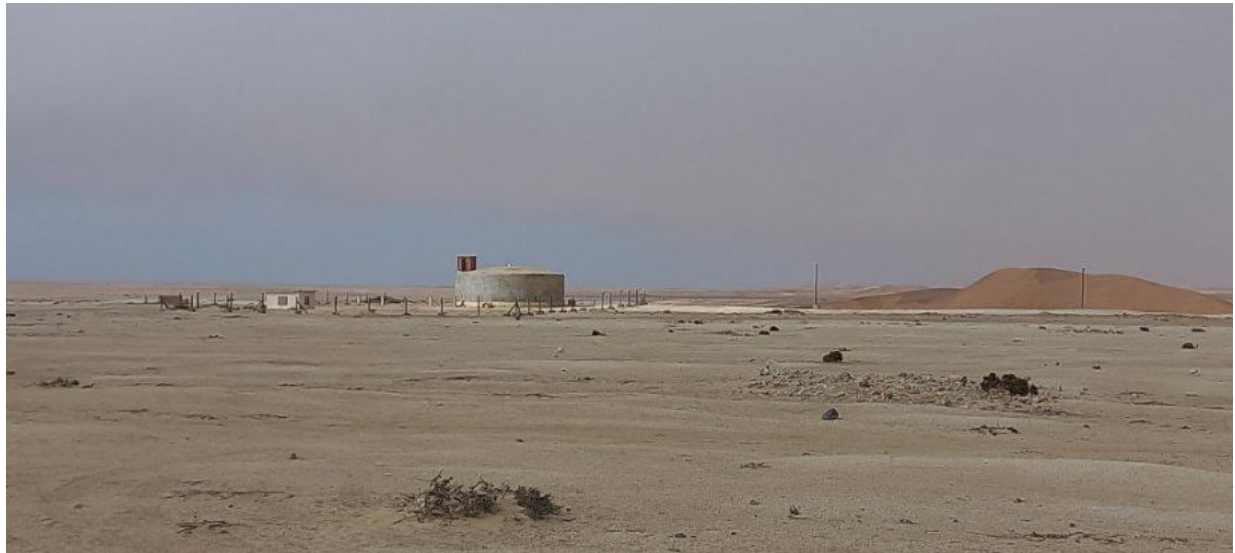
Photo 1.3-3 – South-easterly view of the bulk water reservoir located to the south-eastern side, outside of Extension 32 Township.
