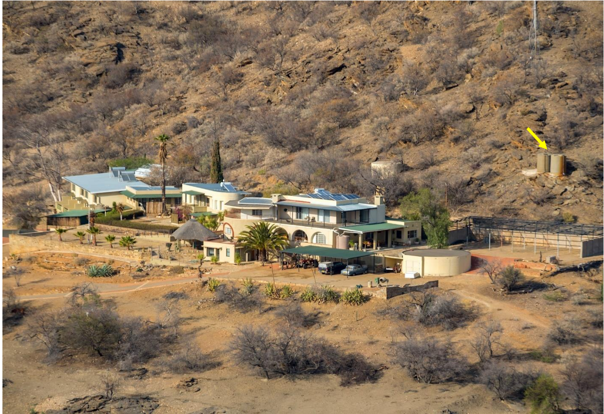
Figure 6: Picture showing the Kappsvalley Lodge and main house, as well as the two 5,000 litre water tanks (Source: Kapps Farm Lodge CC).
