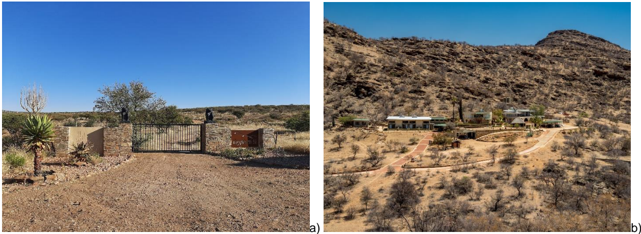
Figure 2: Pictures showing: a) entrance gate to Kappsvally Lodge (Source: L. Maartens, 09 June 2020); and b) view of Kappsvally Lodge (Source: Kapps Farm Lodge CC).
