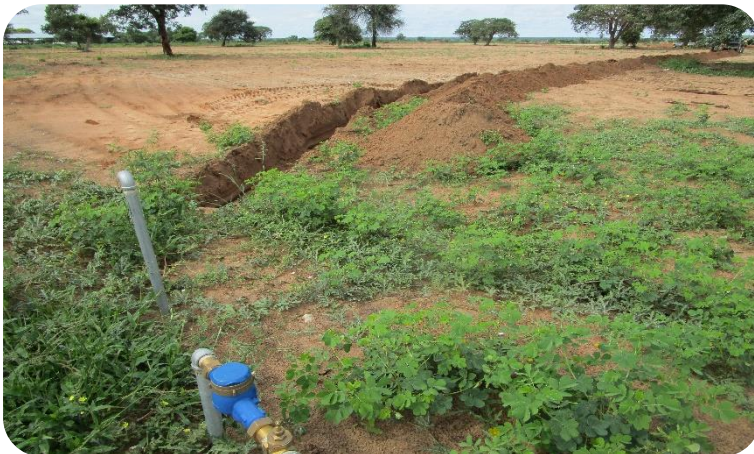
Plate 4: Portable water connection made to the existing bulk water services
