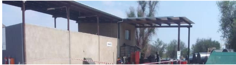
Figure 5. Erection of steel roof over filter draining
