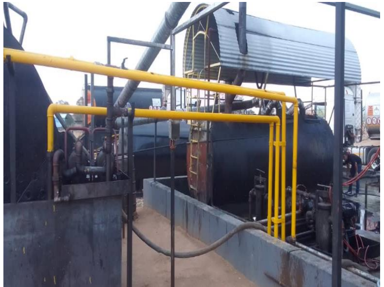
Figure 7. Painting of boiler LFO outlet lines and safety signs
