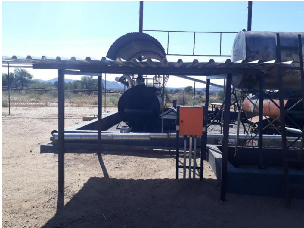
Figure 6. Erection of steel roof over electrical point station at boilers
