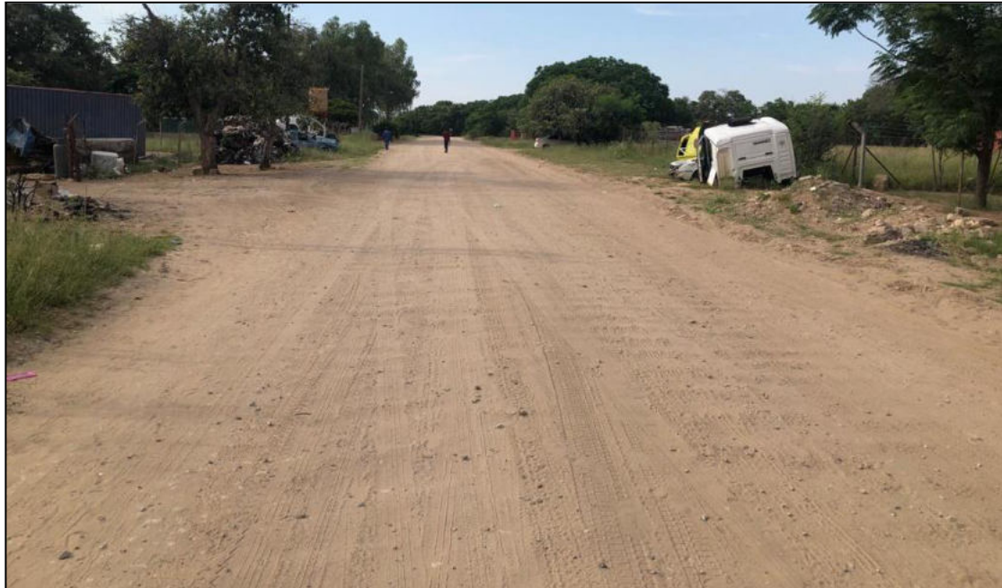
Figure 10: Access road to Project Site
