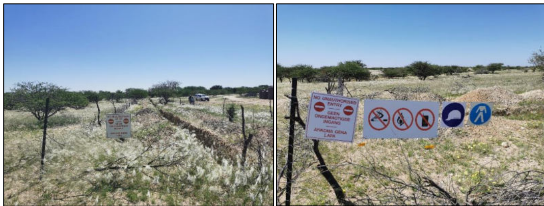
Figure 2-3: Fenced off exploration trenches awaiting backfilling upon completion of sampling at an EPL
