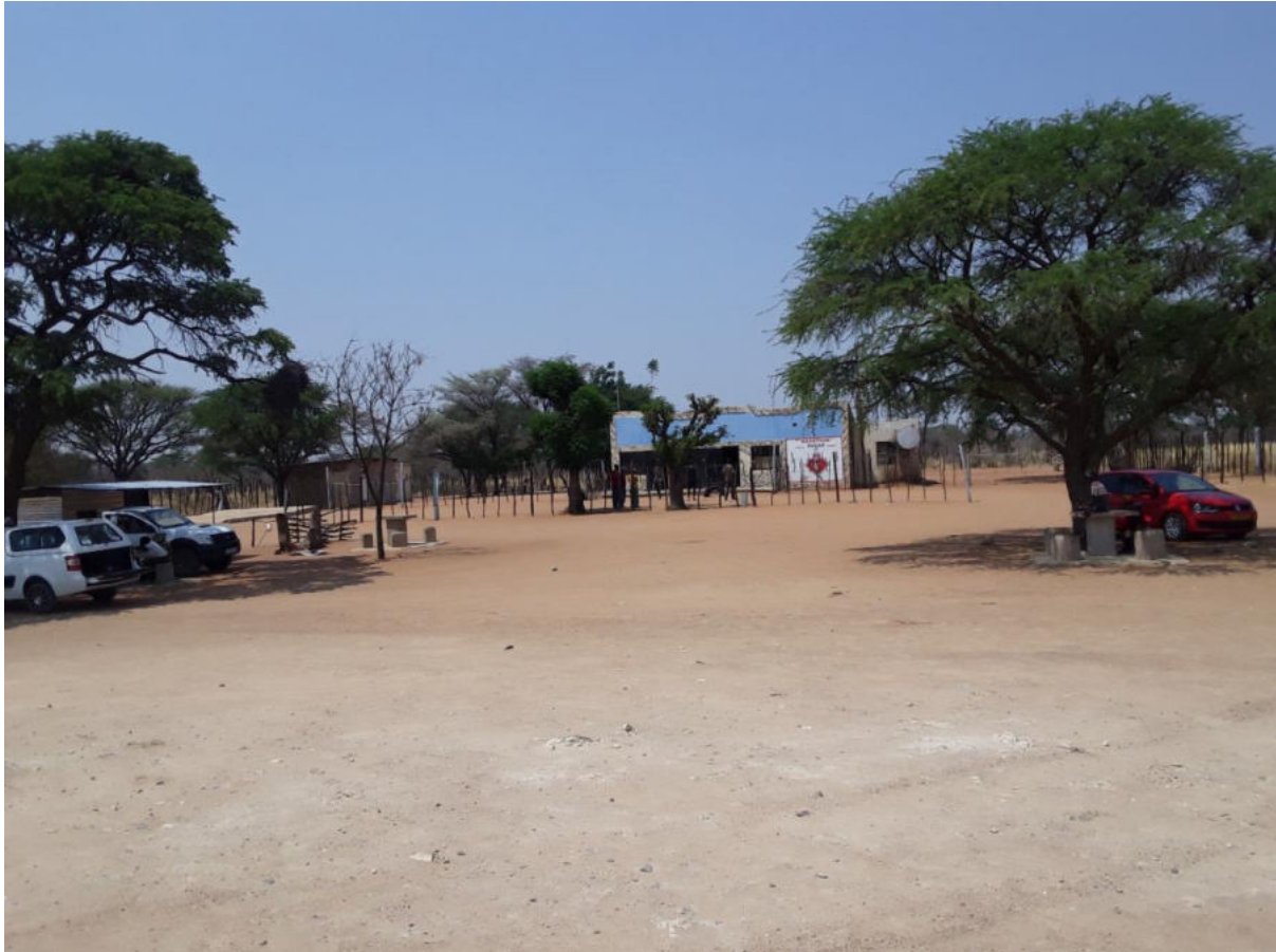
Figure 1 Existing infrastructure of the proposed service station (existing retail shop with a bakery behind, toilets and take away)
