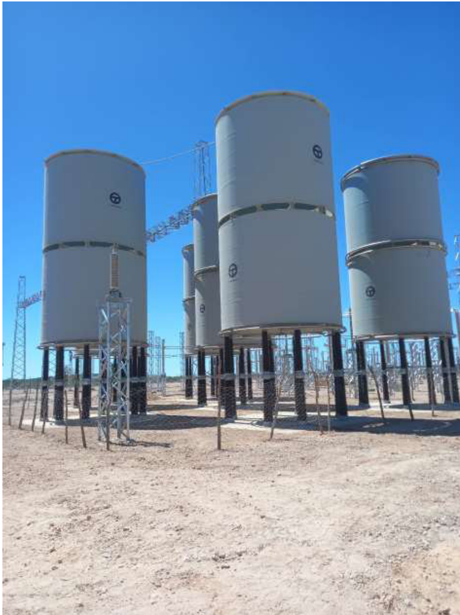
Figure 3: Air cooled reactors installed.
