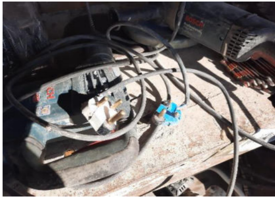
Damaged electric plug
