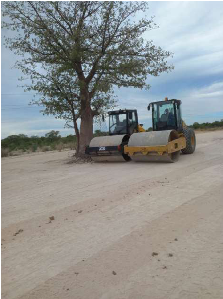
Figure 2 : Rollers during early stages of the project.
