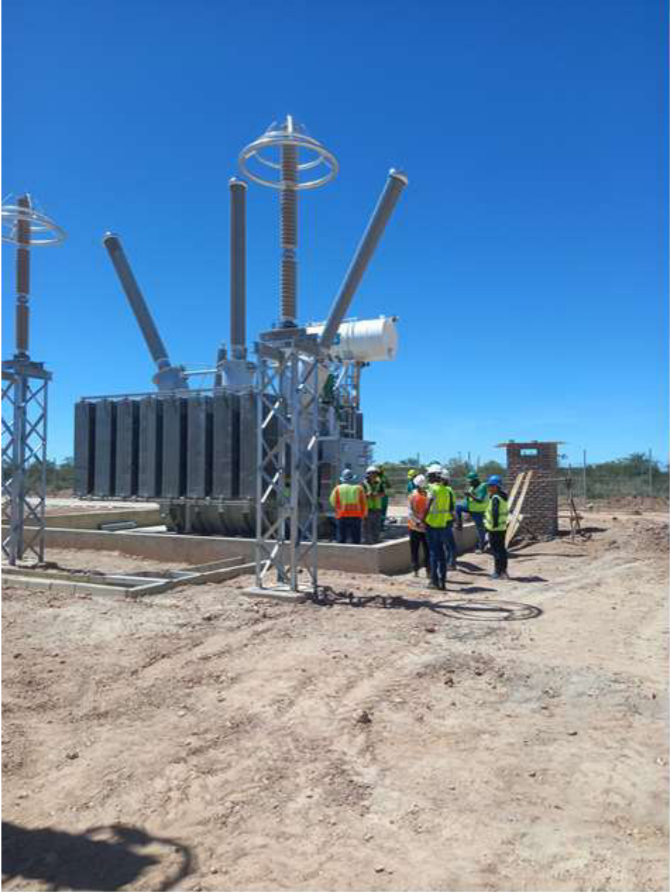
Figure 4 : Project team conduction progress site inspection and overall compliance onsite.
