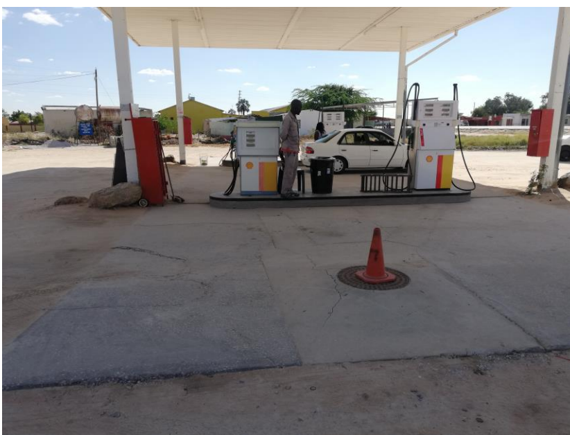
Figure 3. The concrete forecourt
