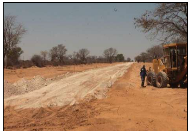
Figure 6: DR3446 Upgrade Underway
