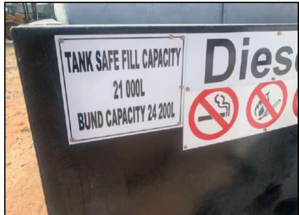
Figure 4: Tank Safe Fill and Bund Capacities
