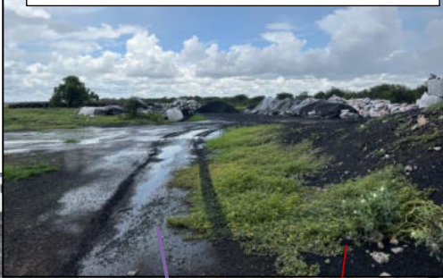
Open charcoal fines storage facility
