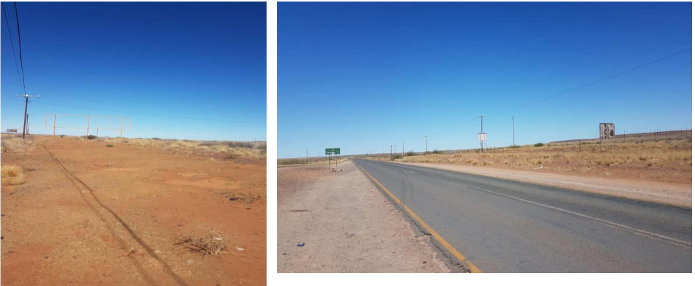
Figure 2: Powerline on project site and B39 road
