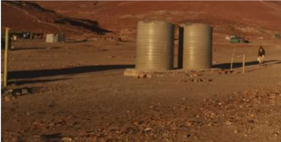
Figure 9: Water Storage tanks at Farm Goboboseb
