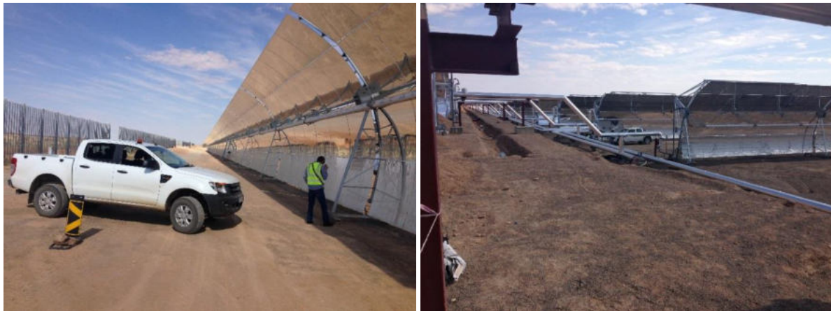
Figure 6: Photographs of the KaXu CSP facility, South Africa
