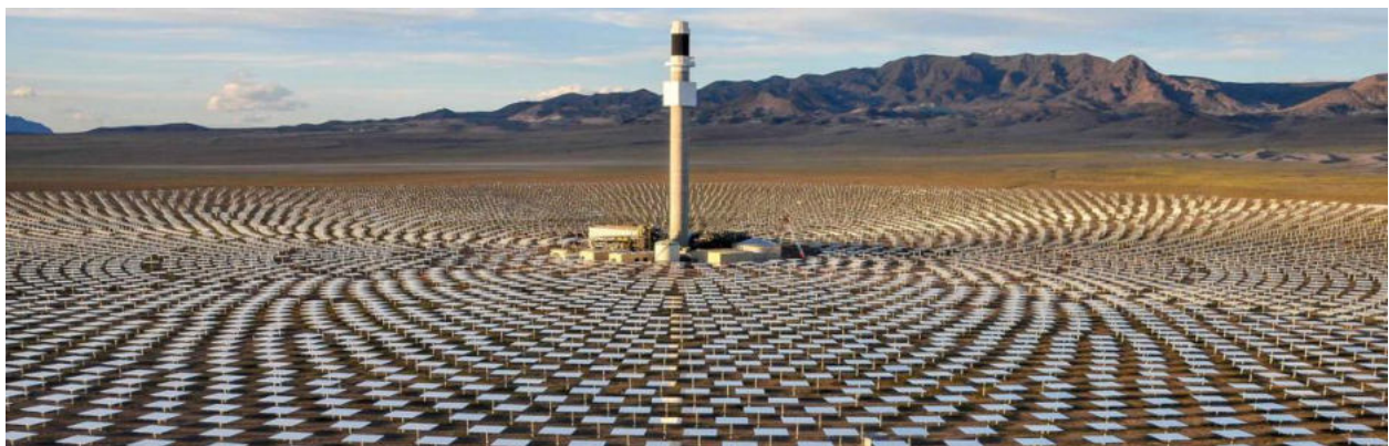
Figure 10: SolarReserve's Crescent Dunes CSP Project, near Tonopah, Nevada, has an electricity generating capacity of 110 megawatts. (Source: SolarReserve)
