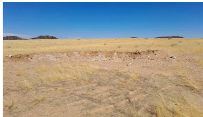
Unrehabilitated small (about 10m wide) borrow pit near the western test quarry. This was used to source material for the adjacent access road
