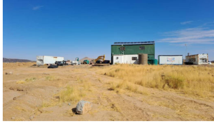
View of exploration camp structures with roof top solar installations for power supply
