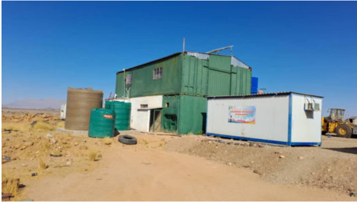
View of main exploration camp structures including containerized offices, accommodation, water supply tanks
