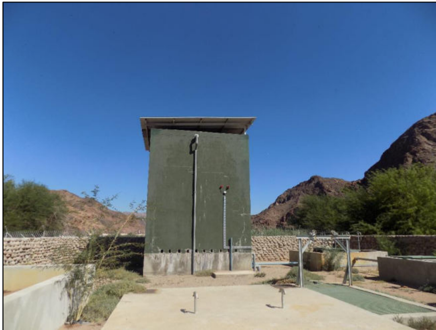
Figure 1-3: Wastewater treatment plant
