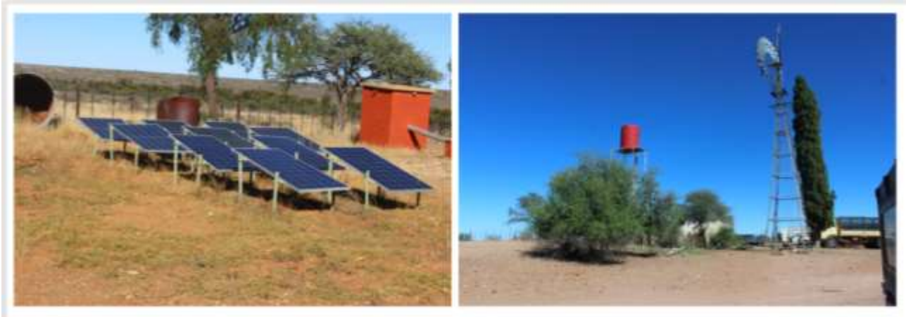
Figure 13: Infrastructure observed on farms - EPL 8813
