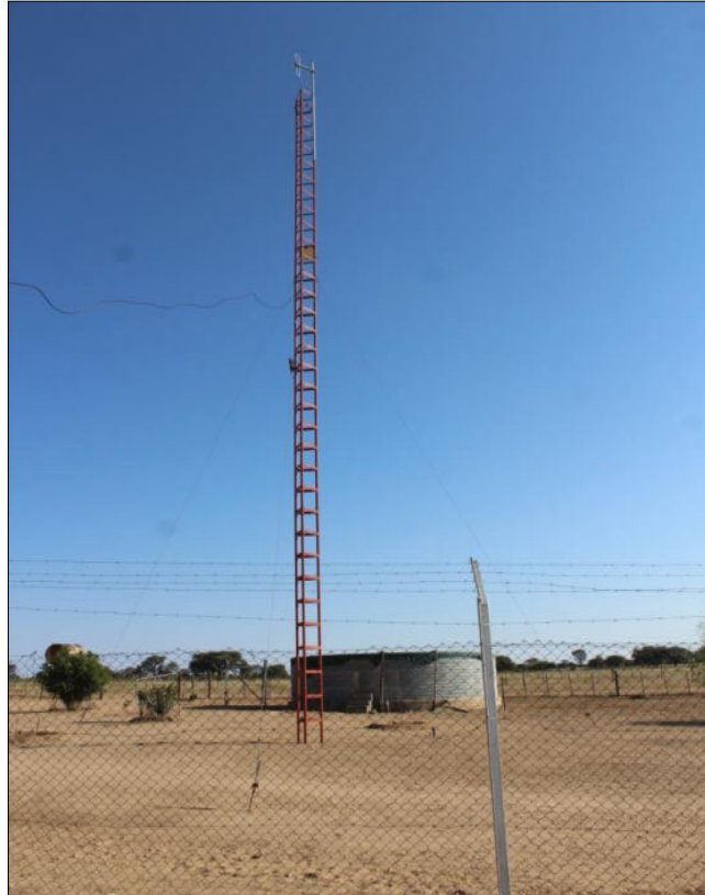
Figure 12: Infrastructure observed on the Farm
