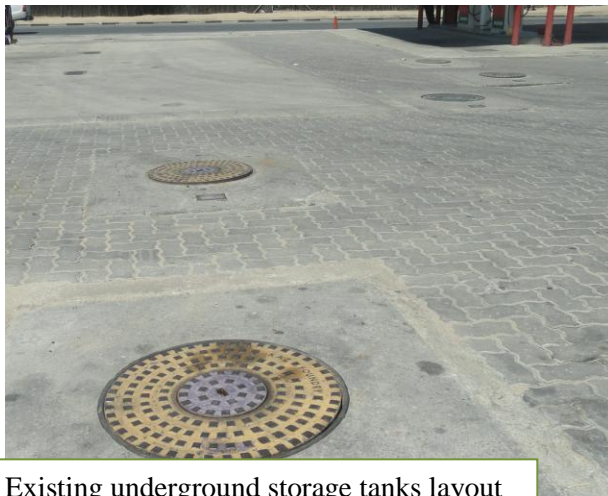
Existing underground storage tanks layout
