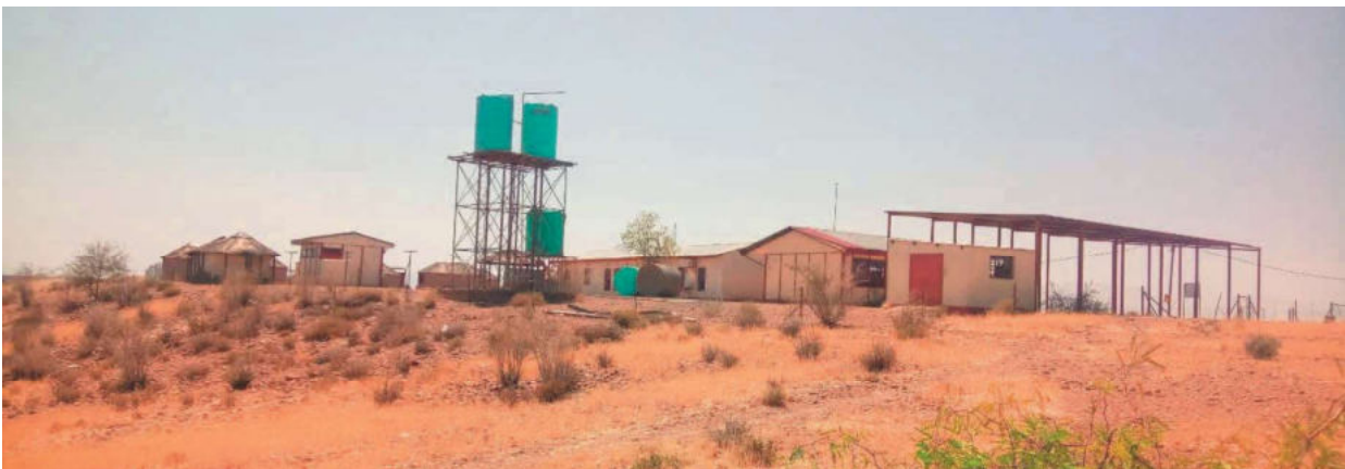
Figure 4: Existing Youth Centre that can be used to accommodate project staff at Kantikoppes settlement
