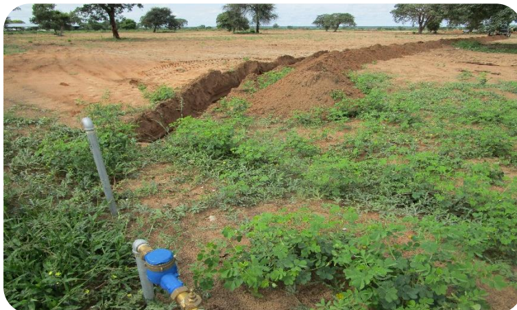
Plate 5: Portable water connection made to the existing bulk water services
