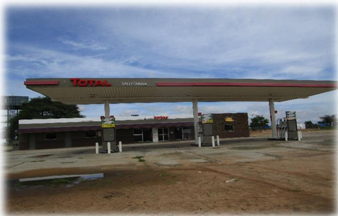
Plate 2: Non-functional Sauyemwa Total filling station
