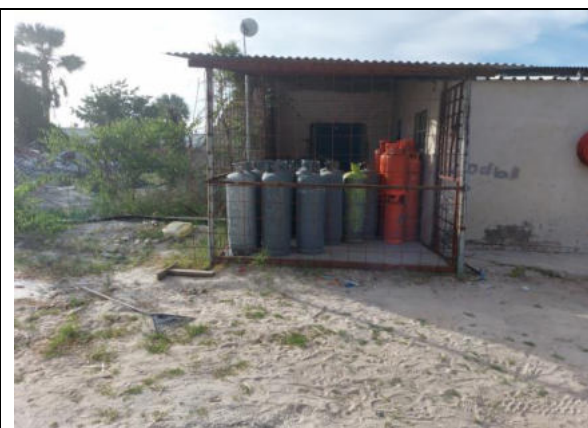
Photo 4-2 LPG cylinder storage area
