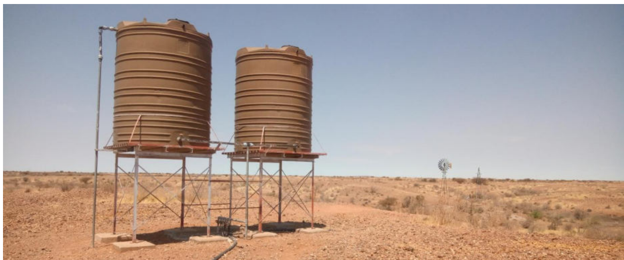
Figure 5: Shows the available water supply infrastructure (forefront, is the tanks and background Windmill)
