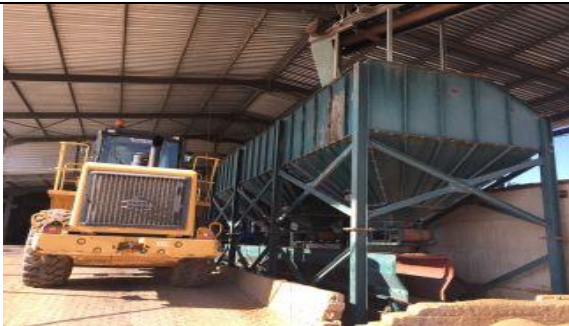
Loading raw material into the automated brick and paver producers
