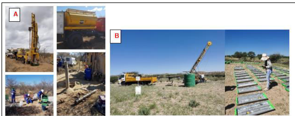
Figure 2-6: A – The common drill rigs for Base & Rare and Precious Metals exploration (Resilient Environmental Solutions, 2019), B- drill rig for Precious Metals exploration site visited in Erongo Region (photo by Author, 2022)
