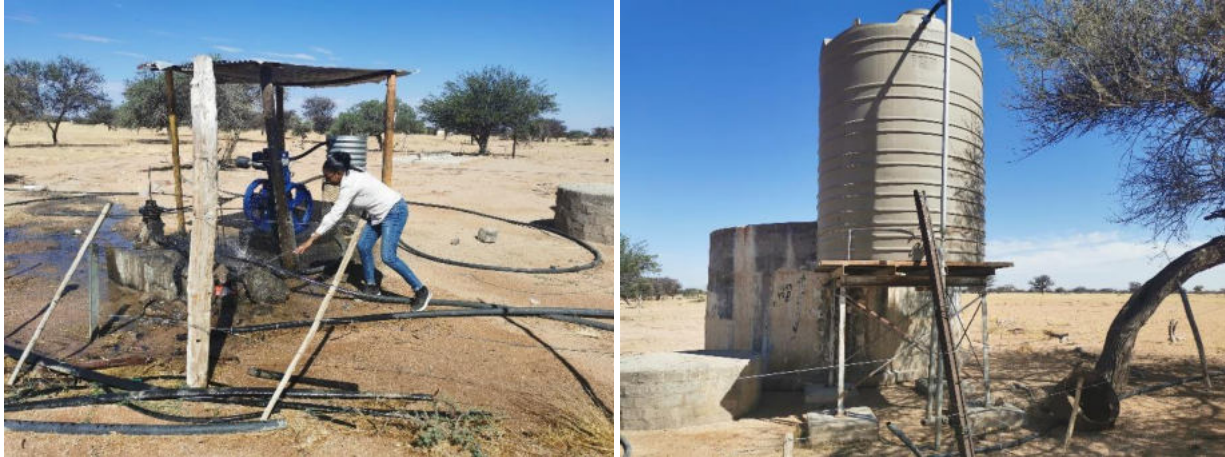
Figure 5-13: The borehole on Farm /Khomxadare and water storage tank
