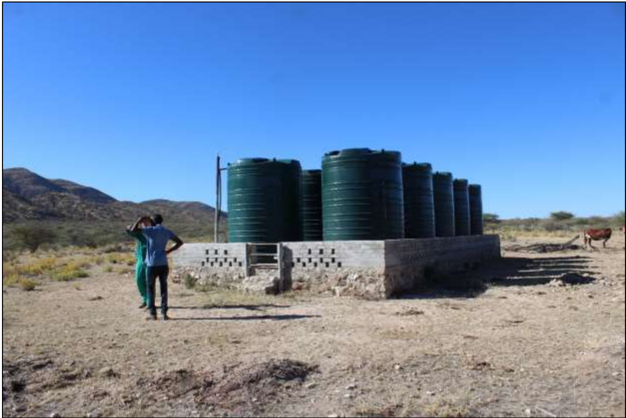
Figure 9: the water tank observed within the EPL
