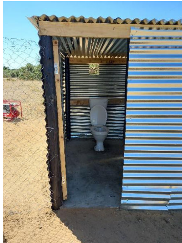
Figure 6 : Toilet at Shiyambi Substation.
