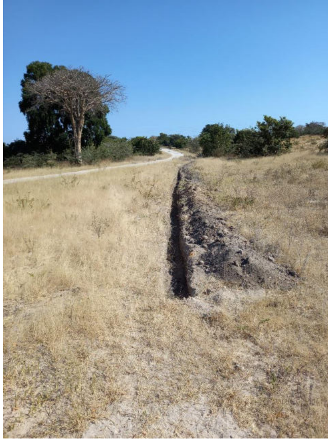
Figure 10: Open Water pipe trench along the Masivi access road.
