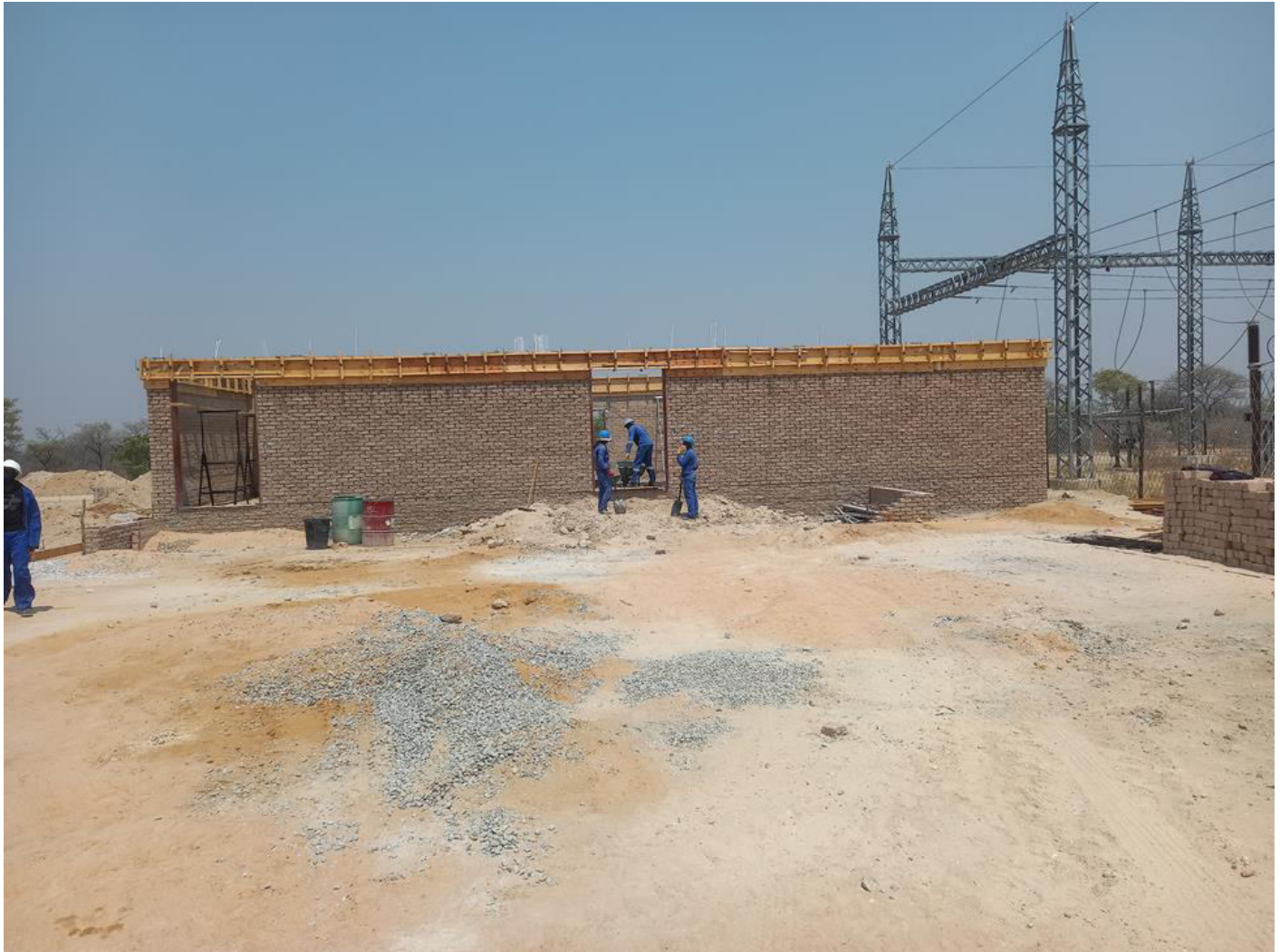
Figure 4: Control building progress at Shiyambi Substation project site.
