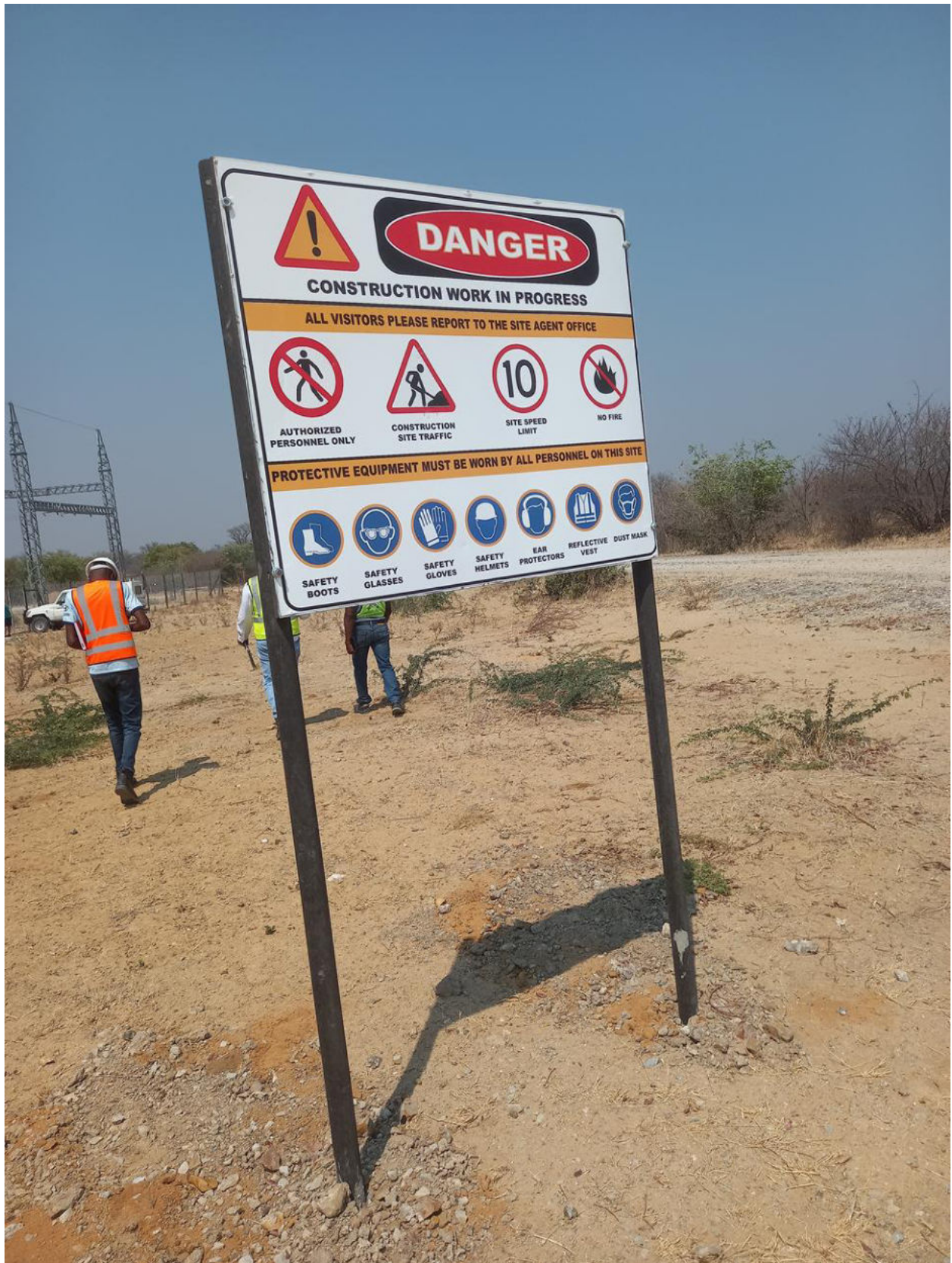
Figure 3 : Signage at Masivi project site.
