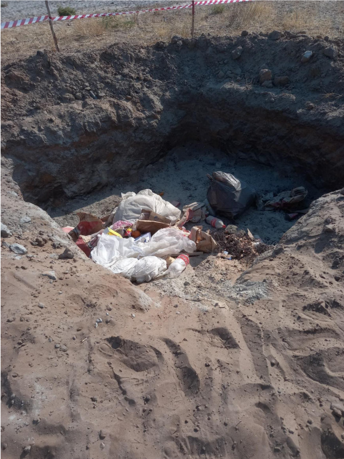
Figure 2: Burning of waste at Masivi project site ( this is prohibited according to the EMP).
