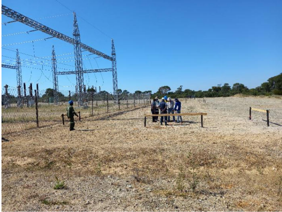
Figure 5: Inspection of setting out at Shiyambi substation.
