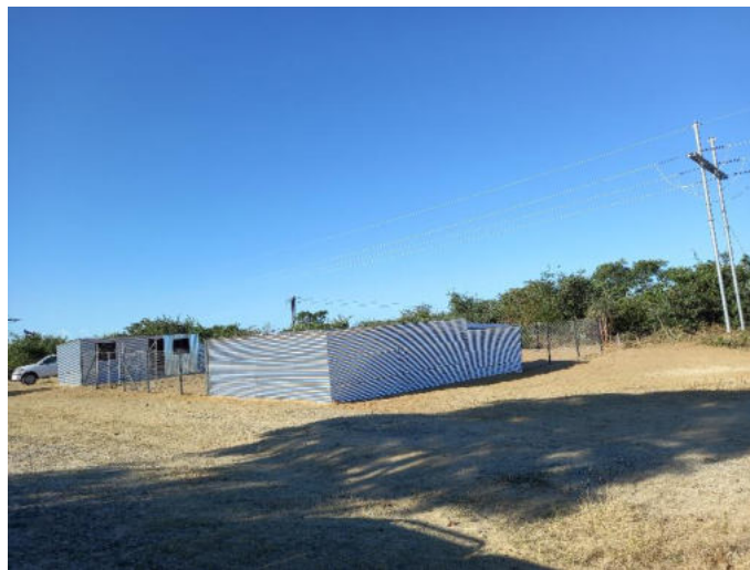
Figure 1 and 2 : Campsite at Masivi Substation and Shiyambi substation.
