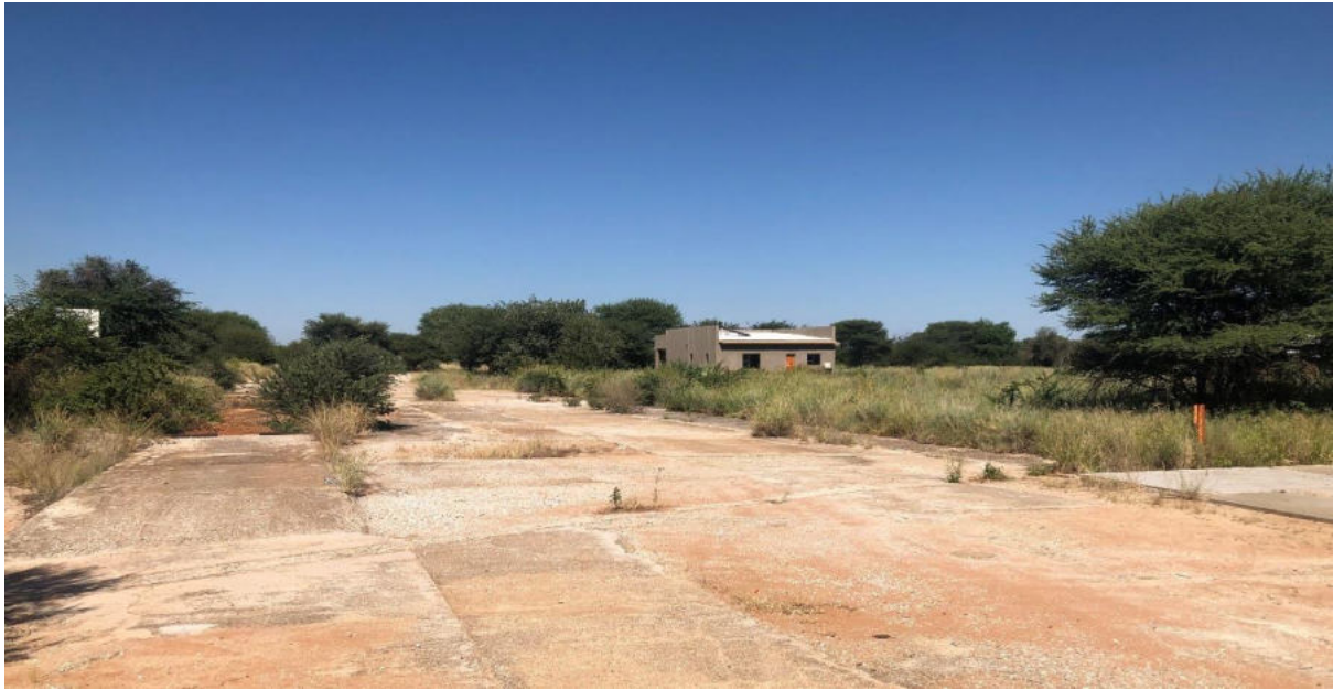
Picture 2 Disused infrastructure within the NIDA Industrial Park
