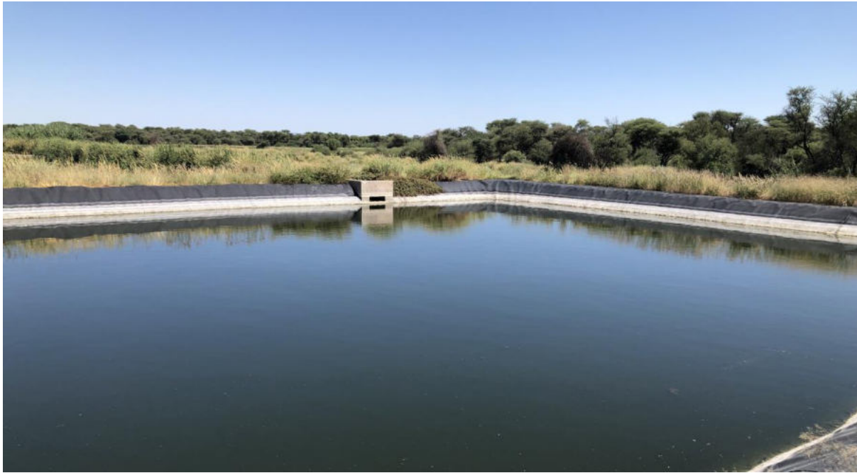
Picture 9 Municipality of Otjiwarongo effluent treatment ponds
