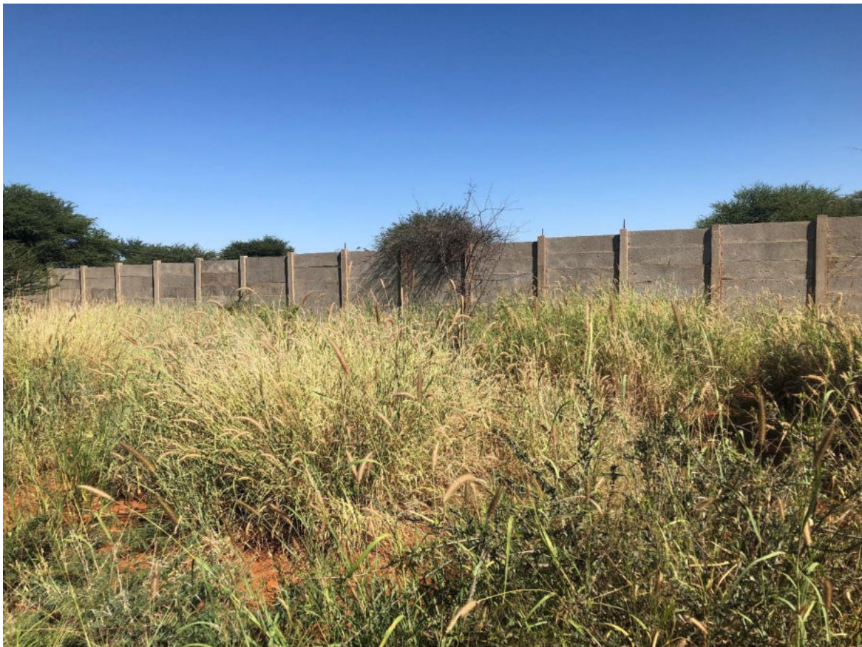
Picture 3 Precast fencing around the NIDA Industrial Park
