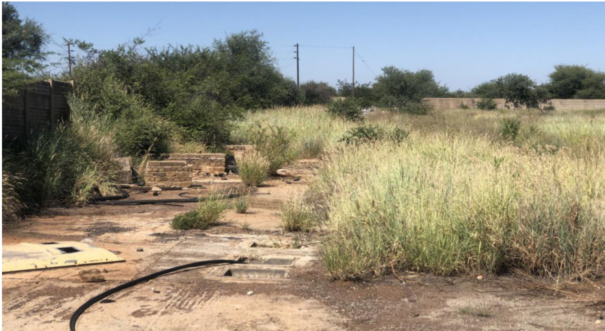
Picture 8 French drain systems on the NIDA Industrial Park premises
