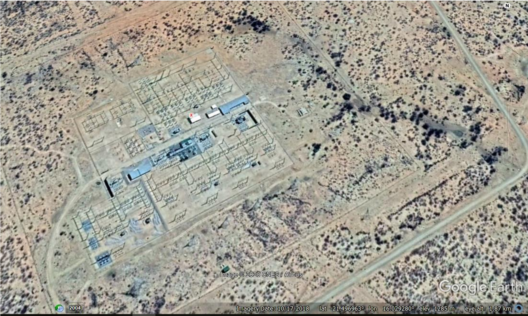
(a) Existing substation.
