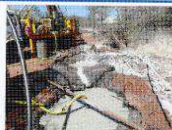
Plastic-lined sump with drilling fluids
