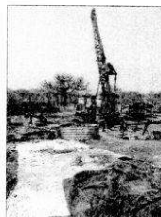
Drill rig and sumps
