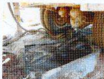
Plastic lining under drill-rig/truck
