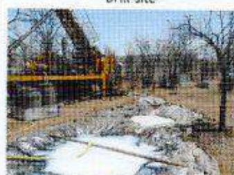
Plastic-lined sumps with drilling fluids
