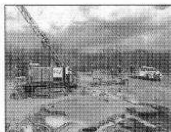
Drill-rig and sumps
