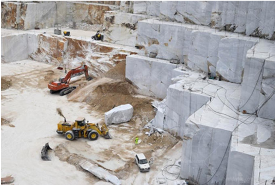
FIGURE 4 - HEAVY MACHINERY USED TO MOVE OVERLYING MATERIAL
