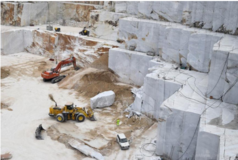
FIGURE 2 - HEAVY MACHINERY USED TO MOVE OVERLYING MATERIAL
