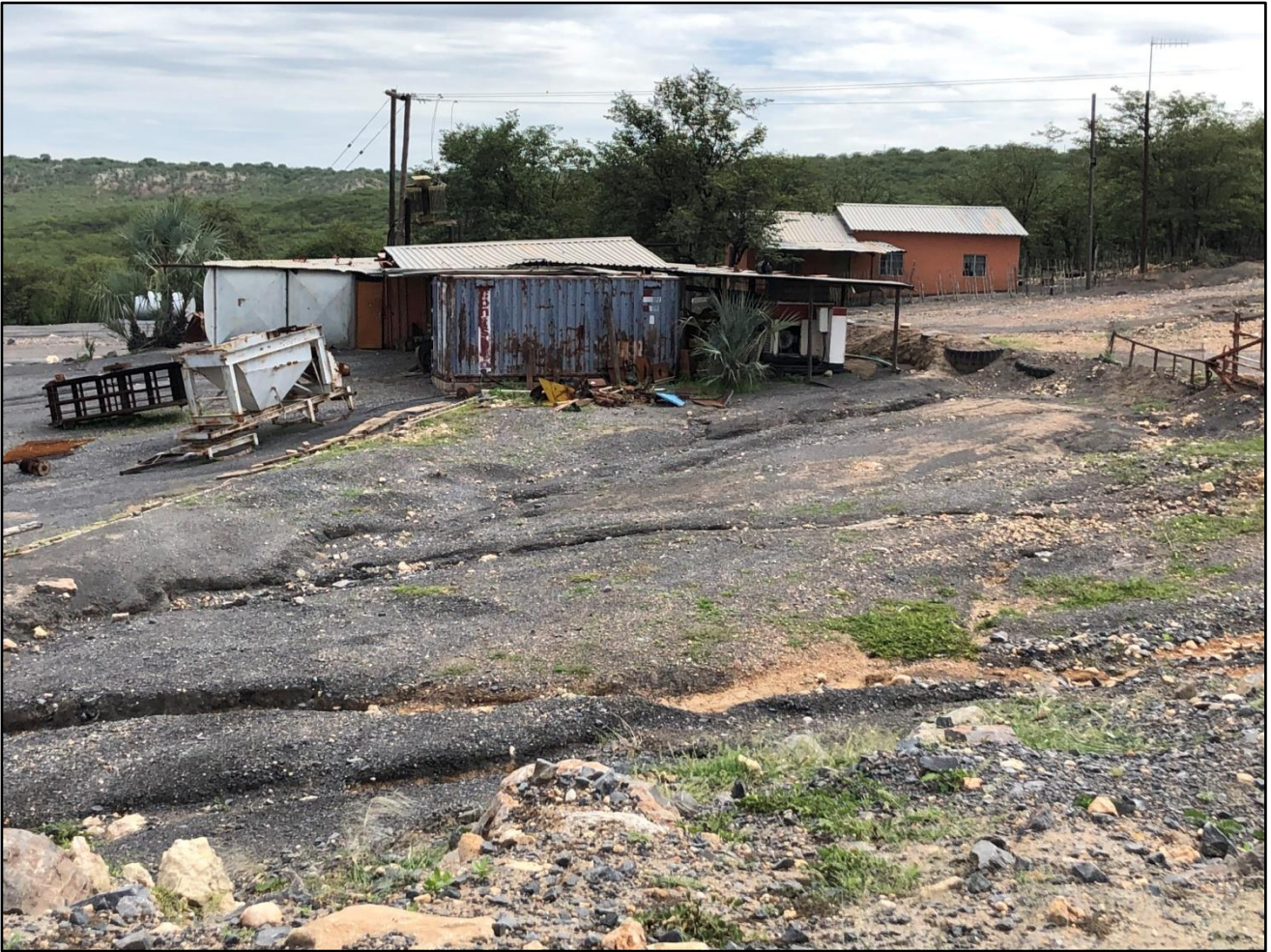
Figure 4: Site workshop (white and grey structure with an overhead power line pole) and workers' accommodation (light orange/pink building)
