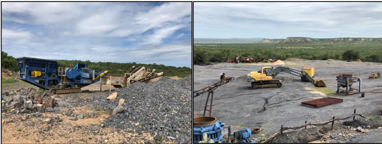
Figure 3: Some of the mining and crushing machinery and equipment on site
