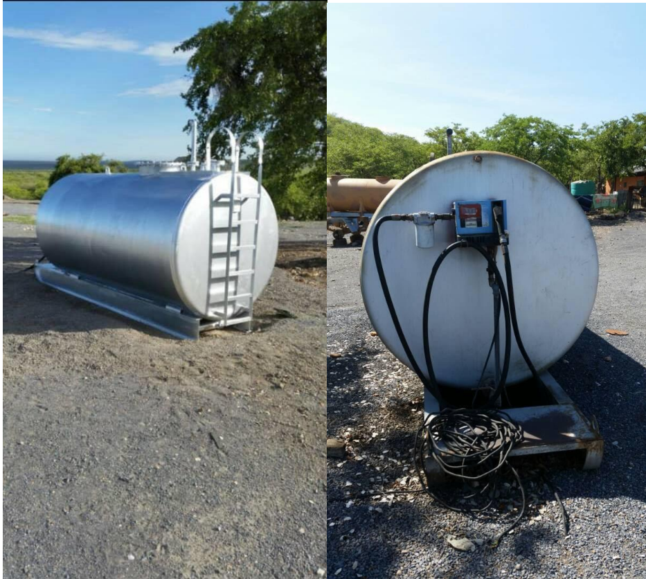
Figure 5: Fuel (diesel) tank on site
