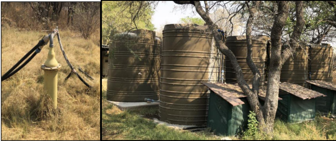
Figure 7: Borehole and water tanks at site
