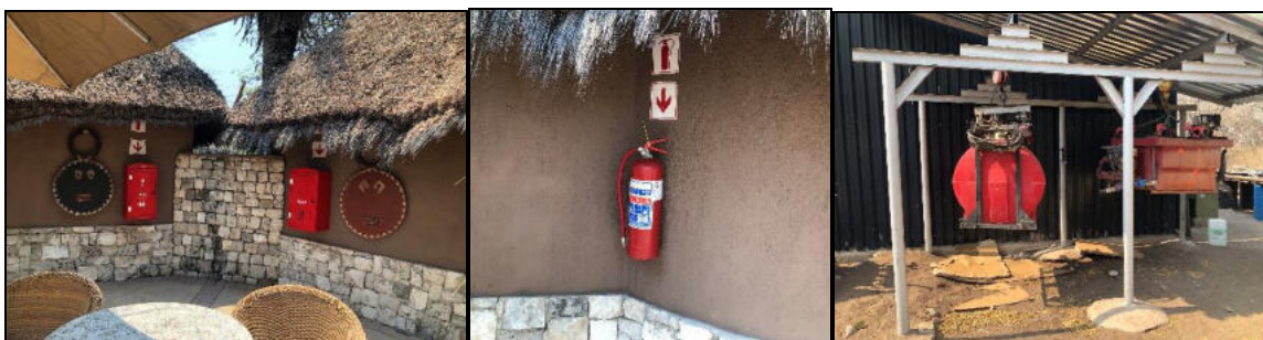
Figure 9: Example of firefighting equipment on site
