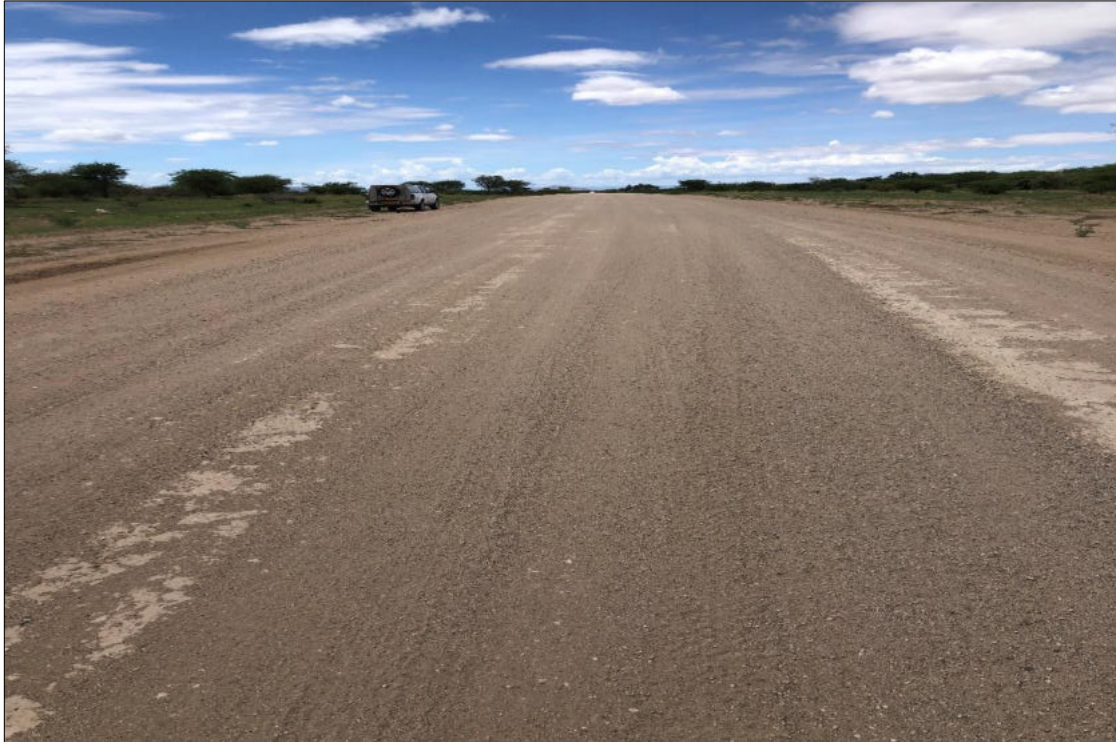
Figure 15: Show a road found within the EPL area
