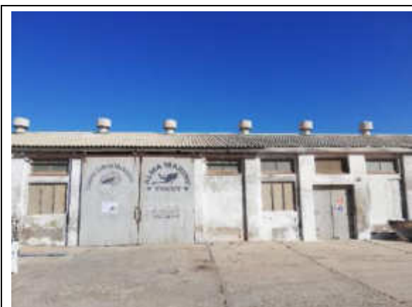
Photo 4-9. Onshore processing facility at Lüderitz Boatyard
