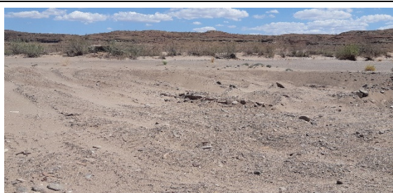
Photo 5. Coarse Material Evened Out Over Mined-Out Area
