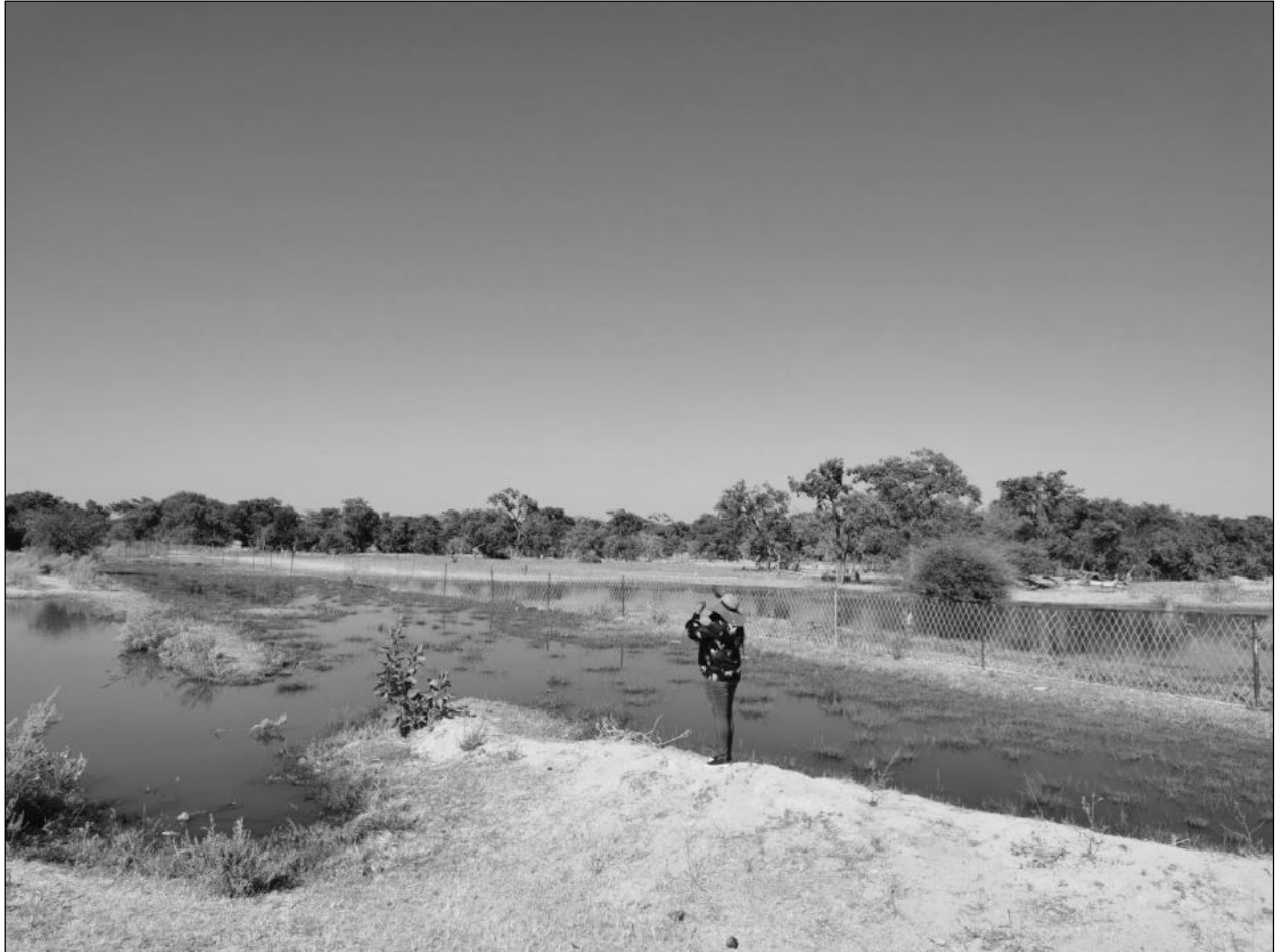
Figure 2-2: The overflowing oxidation ponds towards the western side of the site
