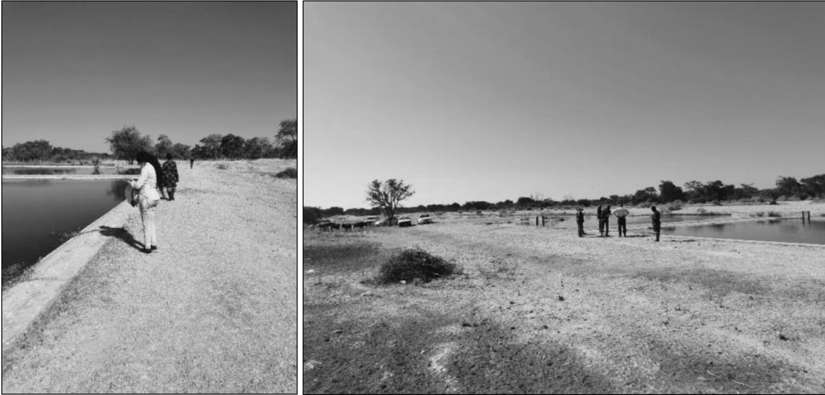
Figure 2-1: The current status of the oxidation ponds on the western edge side of Eenhana Town
