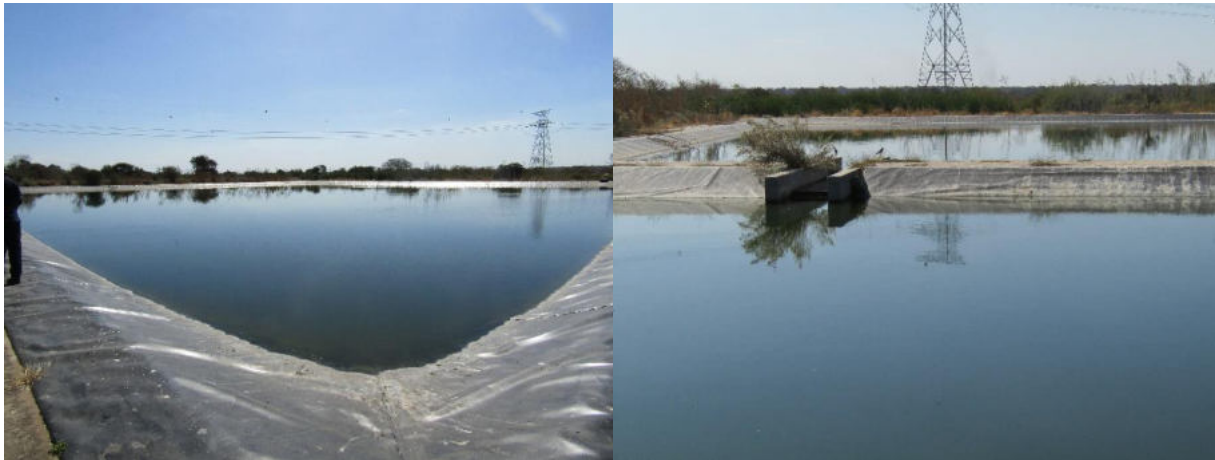
Figure 2-2: The current status of the oxidation ponds in Divundu
