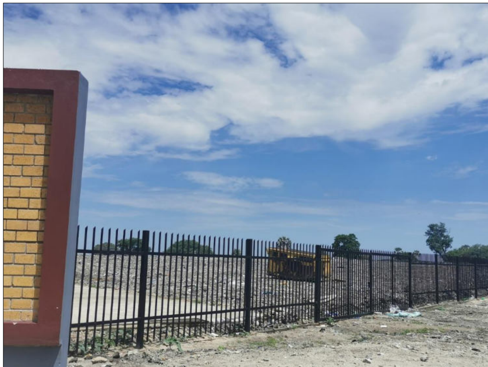
Oshakati Town Council solid waste dumping site entrance and eastern side wall
