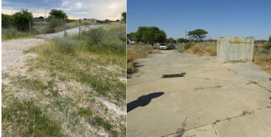
Figure 2-3: The gate at the oxidation ponds' site in Divundu
