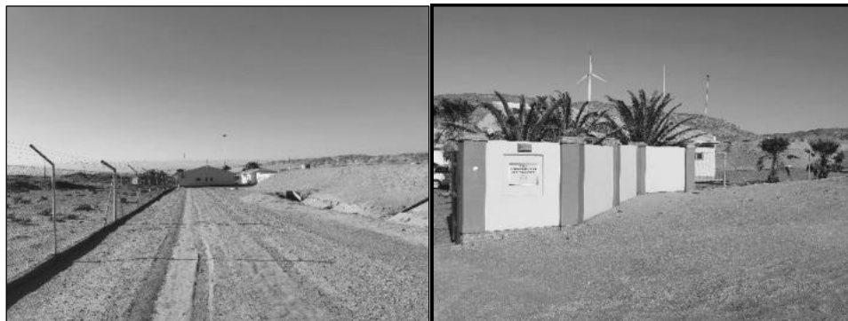
Figure 2-3: The fencing and security around the treatment Plant
