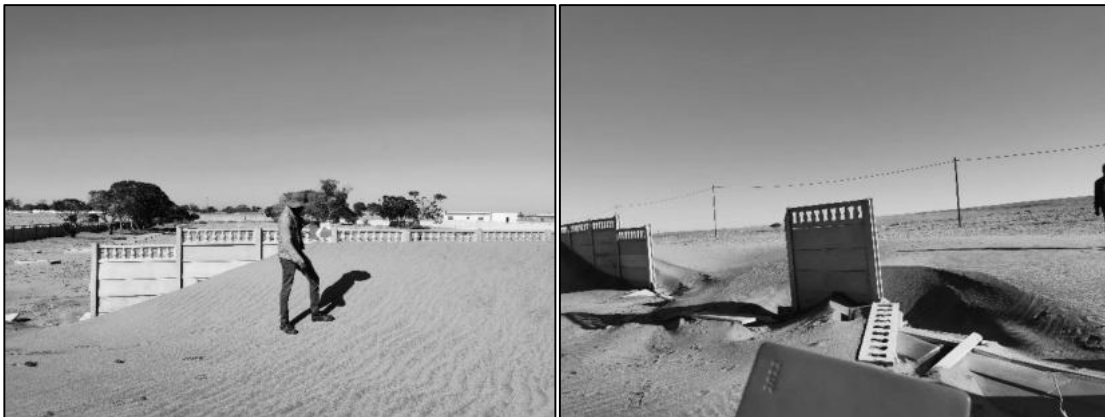
Figure 2-2: The sand accumulation issue at Cemetery Site 2 (immediate west of new cemetery site)
