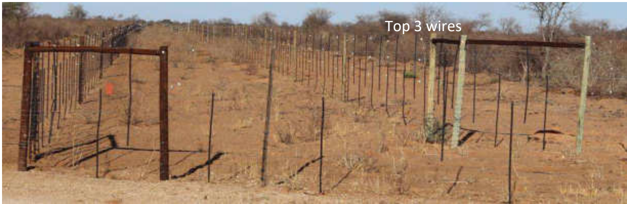
Figure 20: Three (3) top fence-lines with electric fence.
