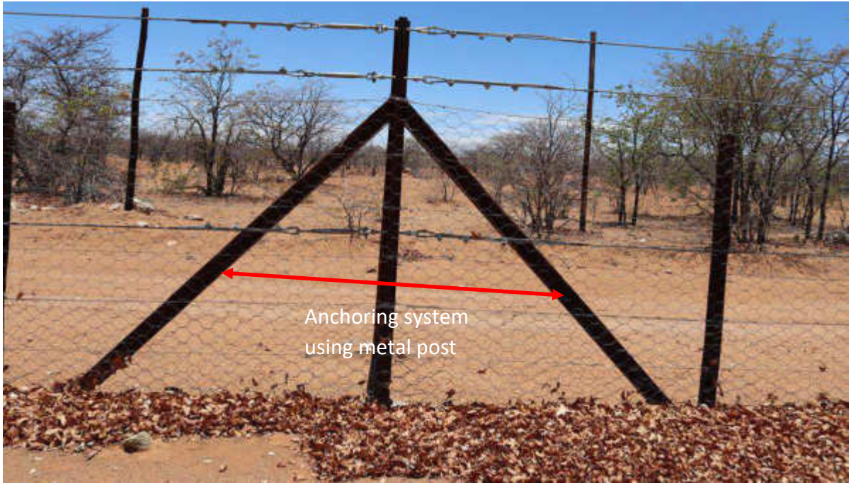
Figure 9: Anchoring system using metal post.
