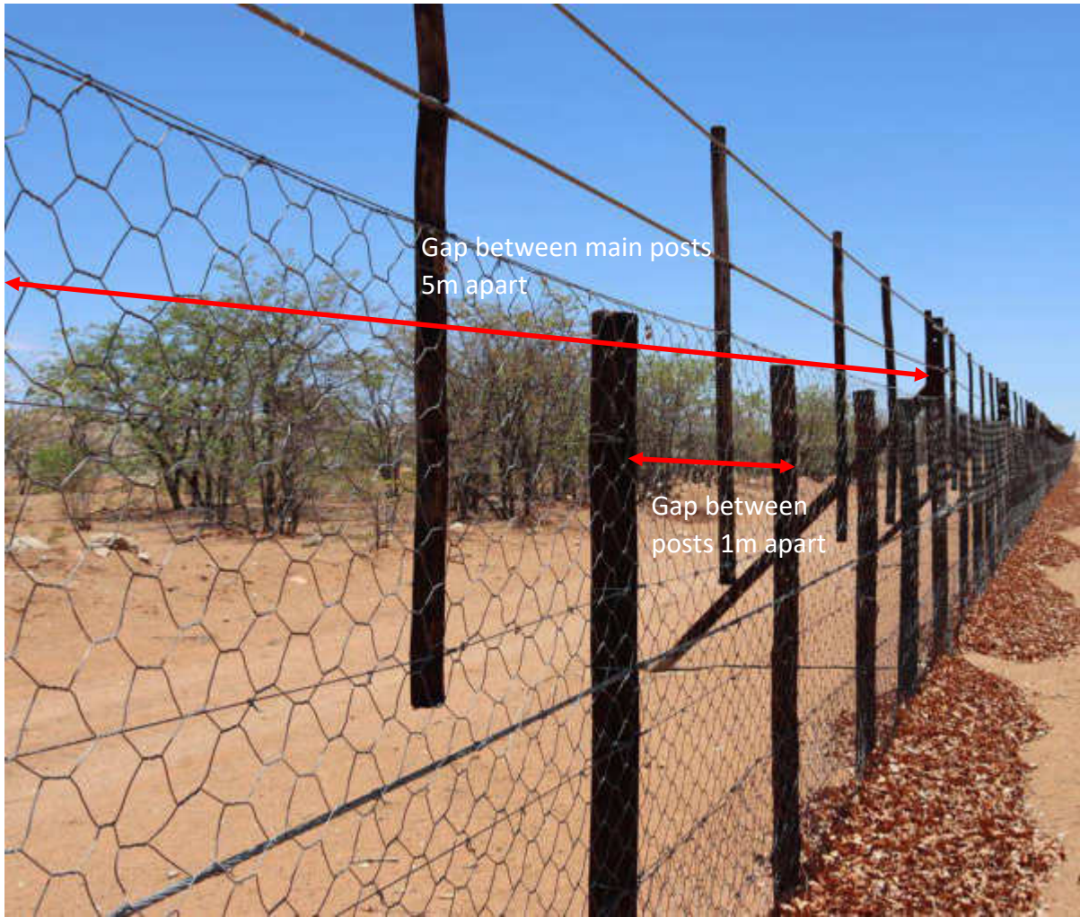
Figure 8: Outer gaps between the posts with 1m apart while main post is 5m apart.
