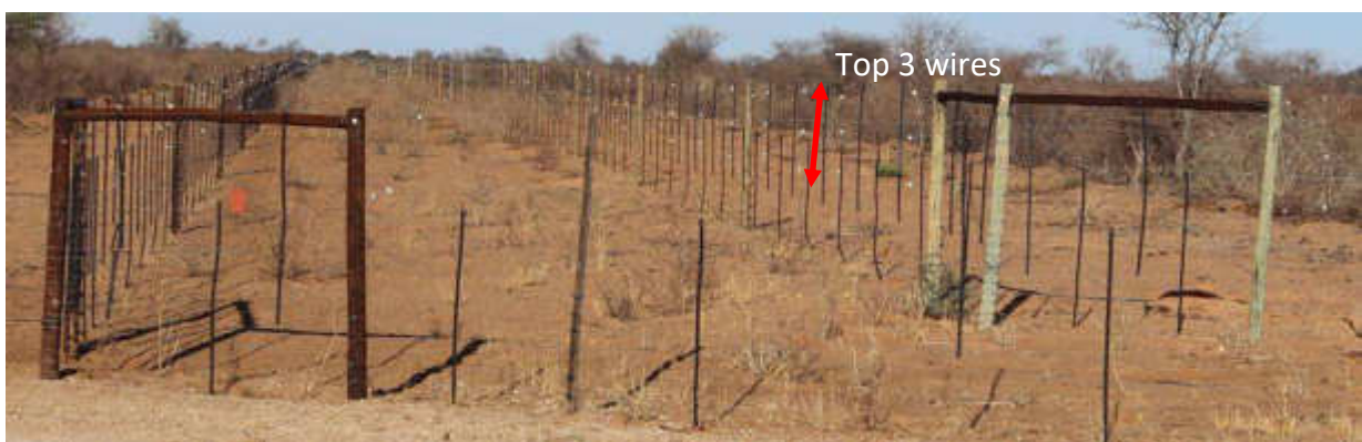
Figure 7: Three (3) top fence-lines with electric fence.
