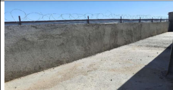
Photo 3-4 Concrete bunding
