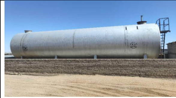
Photo 3-3 Diesel tank
