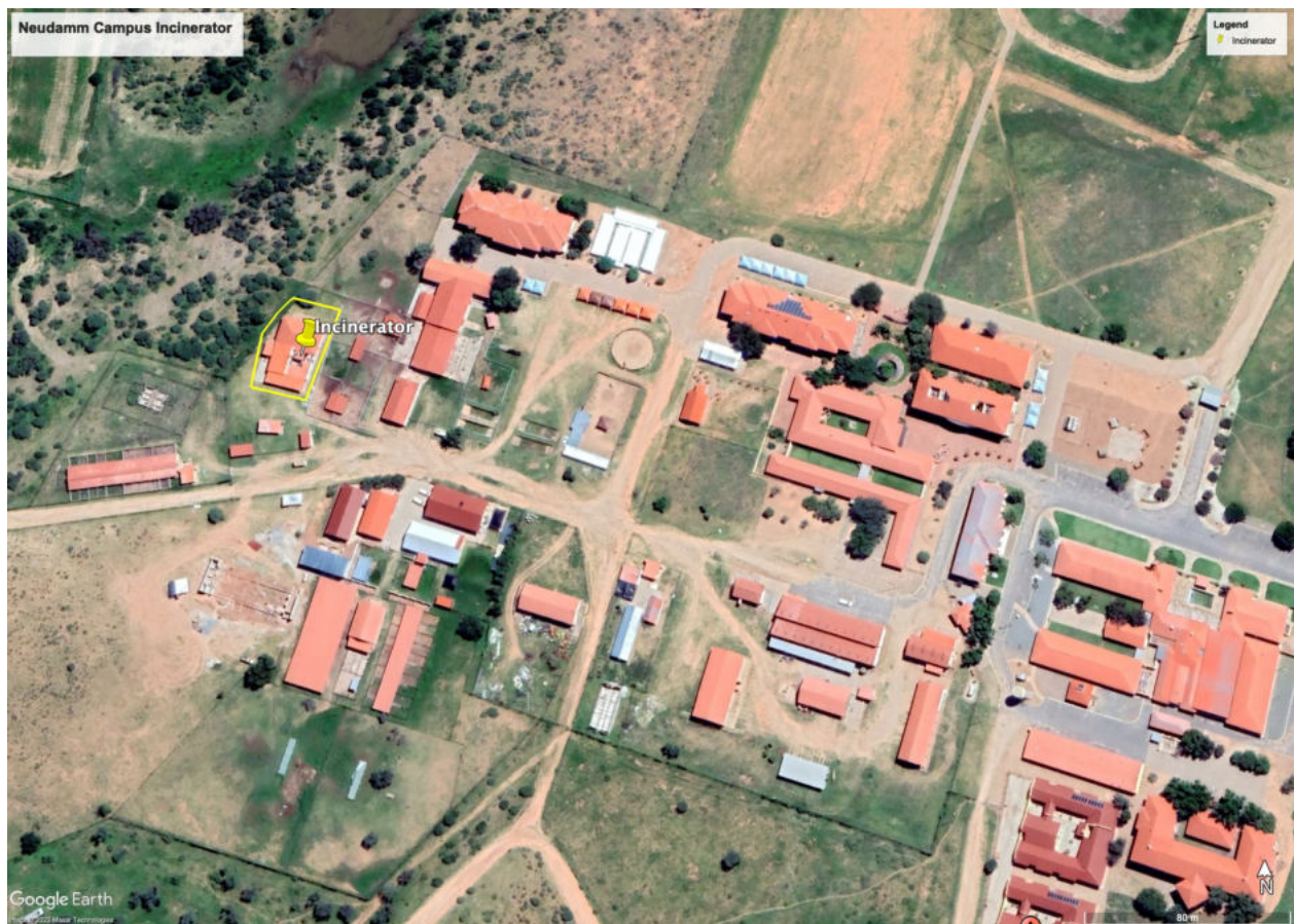
Figure 1. Incinerator at Neudamm Campus
