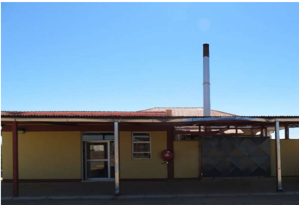
Figure 3. The incinerator building
