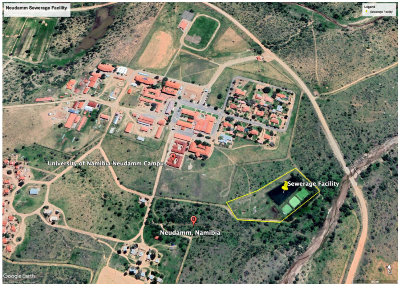
Figure 1. Neudamm Sewerage facility
